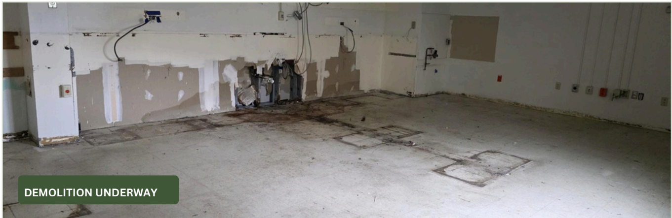
Demolition is underway as the first-floor space is prepared for the future pharmacy.
