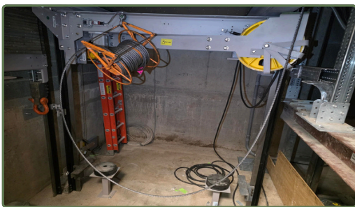
Elevator modernization is upgrading critical equipment that supports reliable access throughout WCHC's five-story campus.
